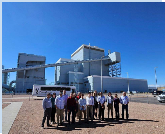
Campbell County Investor Summit attendees gather at Dry Fork power station in Gillette — home to the Wyoming Integrated Test Center and the Wyoming CarbonSAFE project, both sites for carbon capture research.
