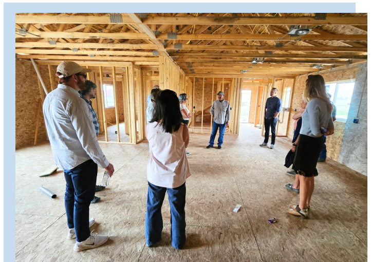
Led by Charles Washakie, Director of Eastern Shoshone Housing Authority, workshop attendees tour a newly built housing development that is planned to receive power from a tribally-owned solar microgrid.
